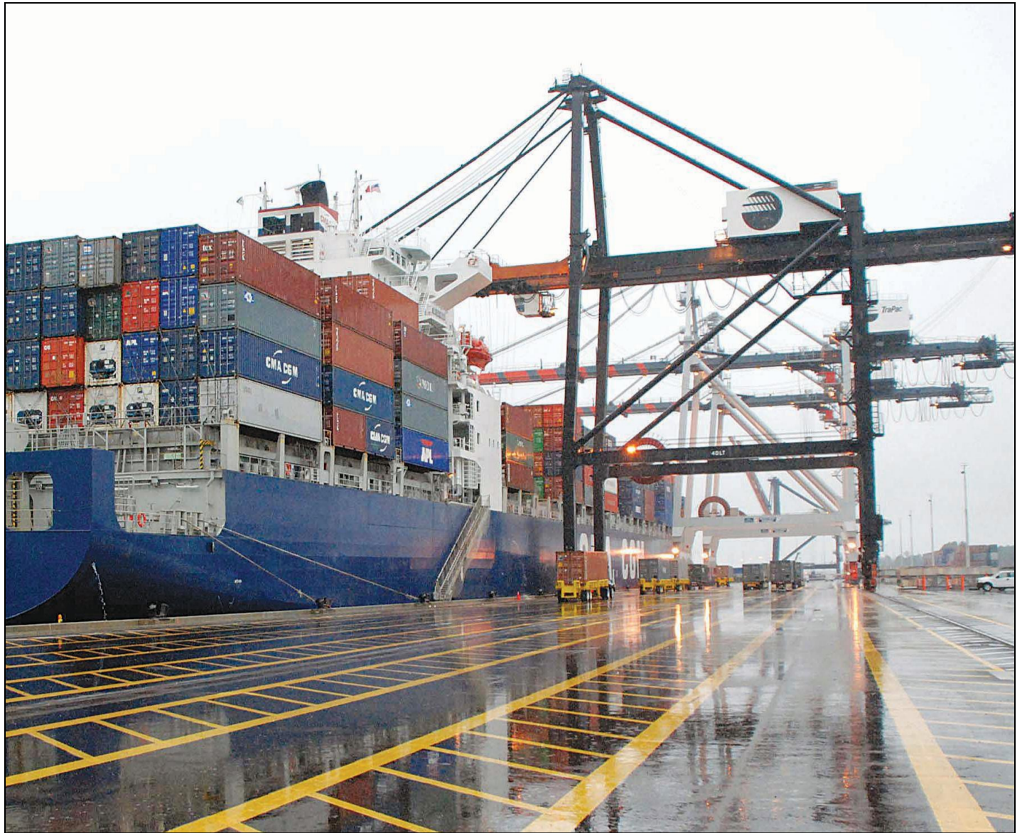
TraPac terminal, Port of Jacksonville, which opened in 2009: volumes have risen since and it is trying to get water depth down to a level that could see post-panamax berth. MOL
